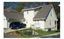
This house on a steep lot has many steps at the front and none at the back. Depending on the lot and house type, a zero-step entrance can be located at the front, back, side or through the garage.
