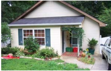
Example: Inexpensive bungalow with sidewalk leading to zero-step entrance
