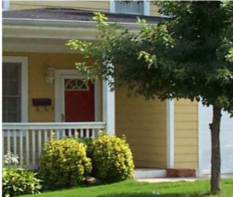
Example: House with small step on the front—hard to retrofit.
